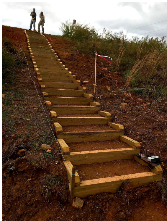
New stairs installed by senior Bracey Fountain
